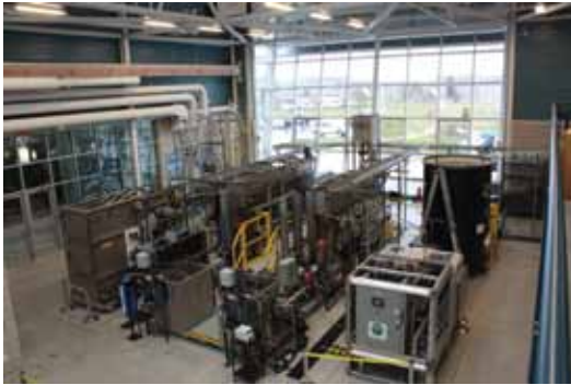
View of the Technology Demonstration Facility.
