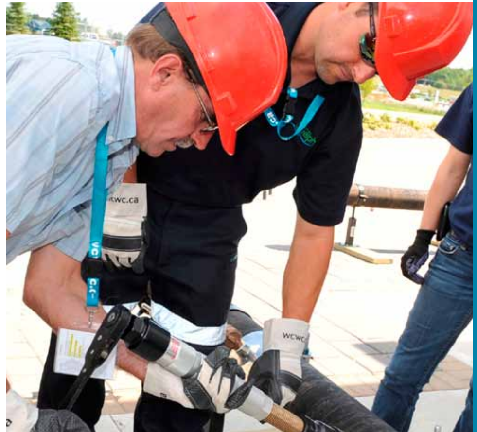
Participants during the hands-on training module, watermain tapping, at the second annual Maintenancefest.
