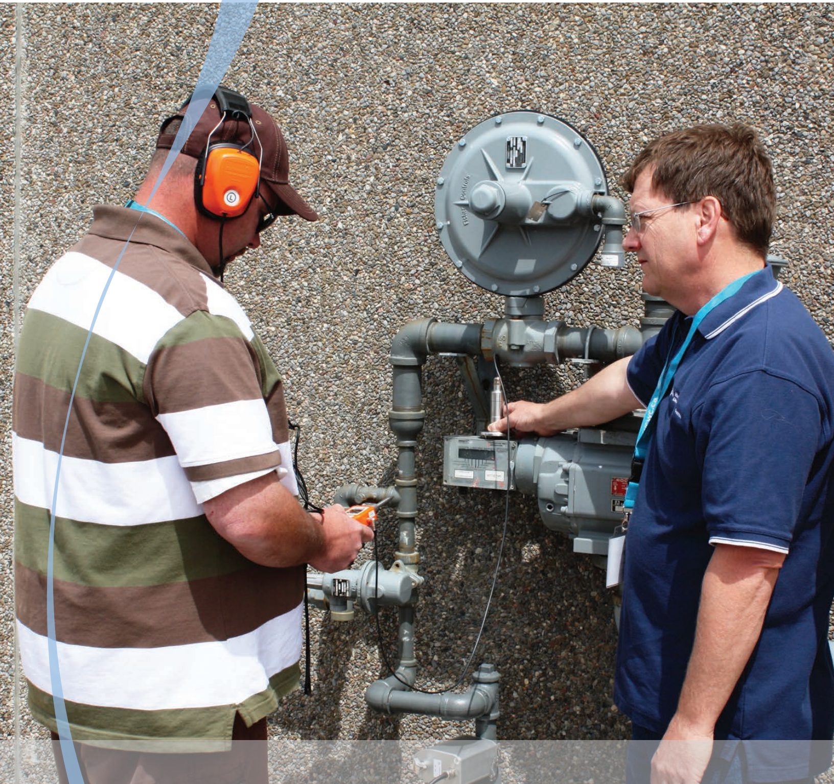
A participant at the regional Maintenancefest event, held in Vaughan, works with a Centre instructor during the Leak Detection Technology and Application module.
